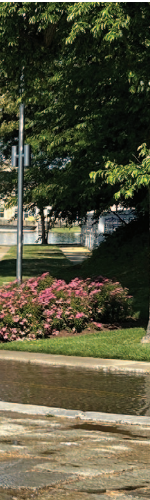
On 3 June, Ramsay Road flooded in front of the Naval Academy Columbarium. It was just one example of nuisance flooding on the Yard minus heavy rains or surging tides.
